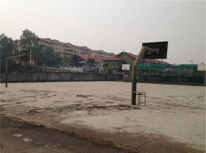
▼ Dilapidated basketball court and sports facilities
